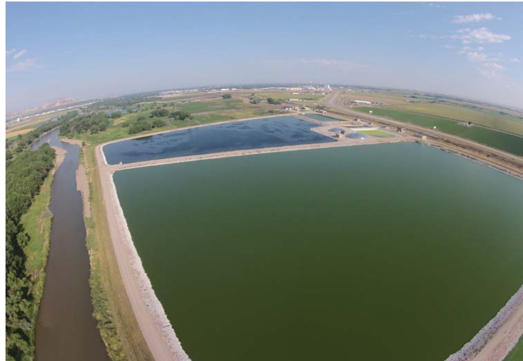
City of Scottsbluff, Wastewater Treatment Plant
