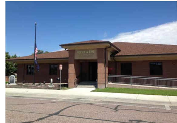
Public Safety Building - West 18th & Avenue B
