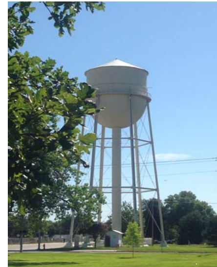
Water Tower - 27th Street & 2nd Avenue
